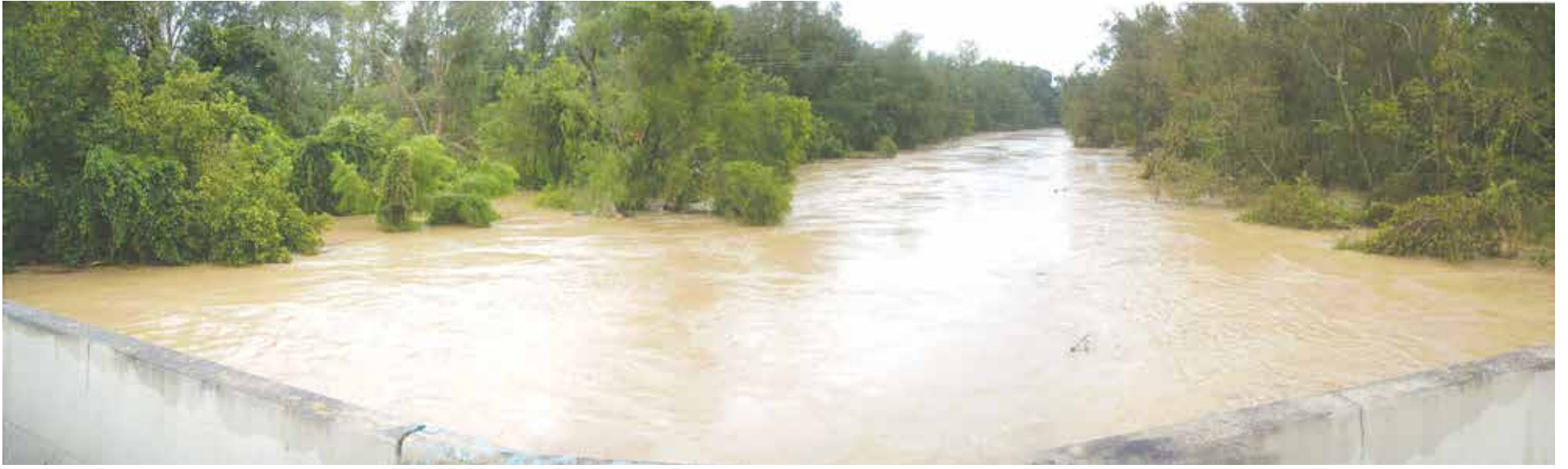
The Comite River, which is the western boundary of the City of Central, overflowed its banks, damaging some neighborhoods during Hurricane Gustav.
