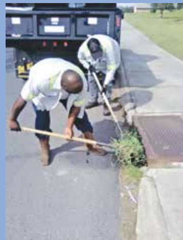
Clearing Clogged Drains
